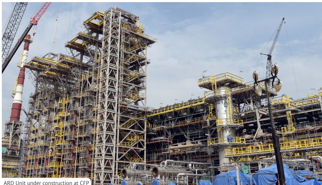
ARD Unit under construction at CFP
