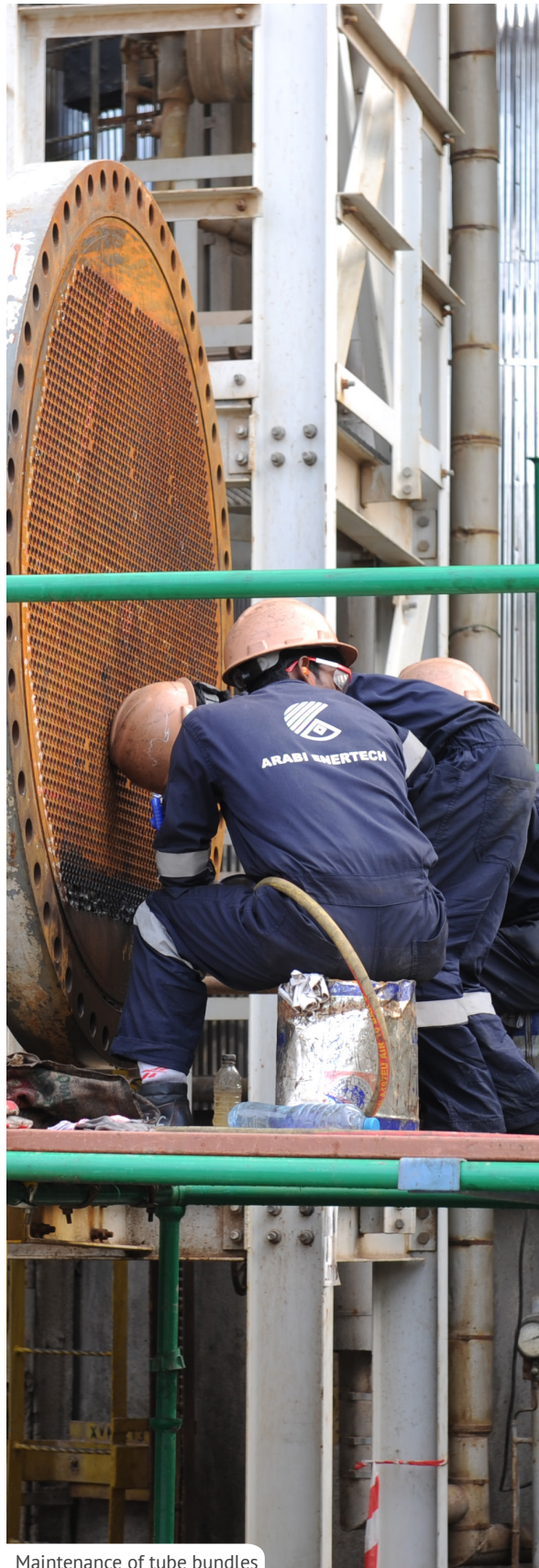
Maintenance of tube bundles
