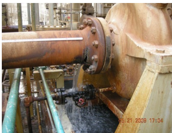
Figure 16a. Perforation of sour water pump
