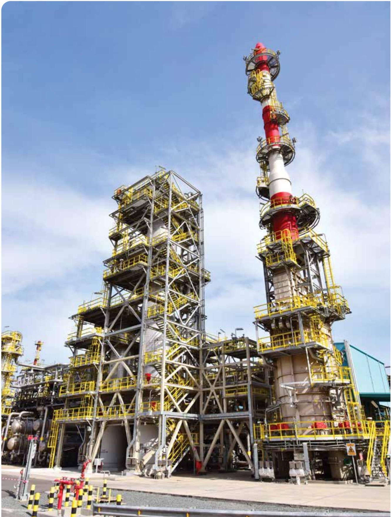
Kerosene Hydrotreating Unit (U-115) - MAB
