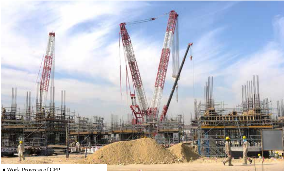
● Work Progress of CFP
