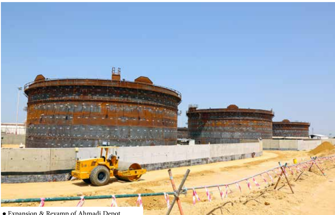
● Expansion & Revamp of Ahmadi Depot
