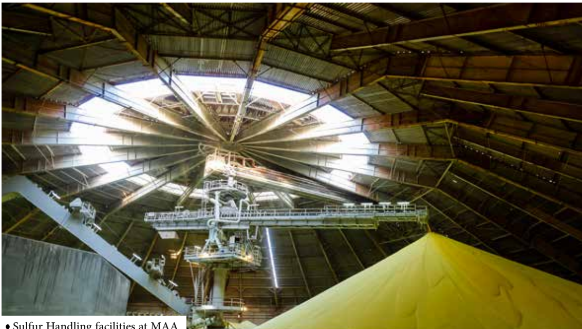
• Sulfur Handling facilities at MAA
