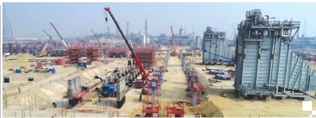
Fifth Gas Train Project
