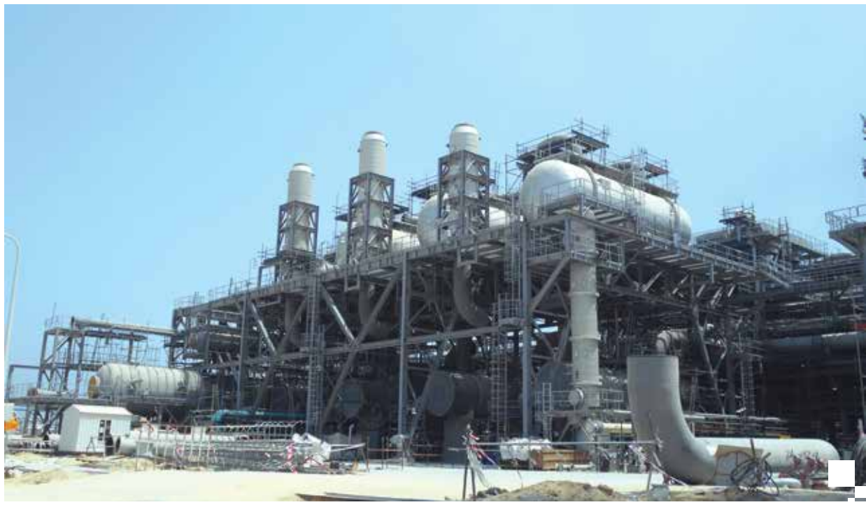
Acid Gas Treatment Unit Project
