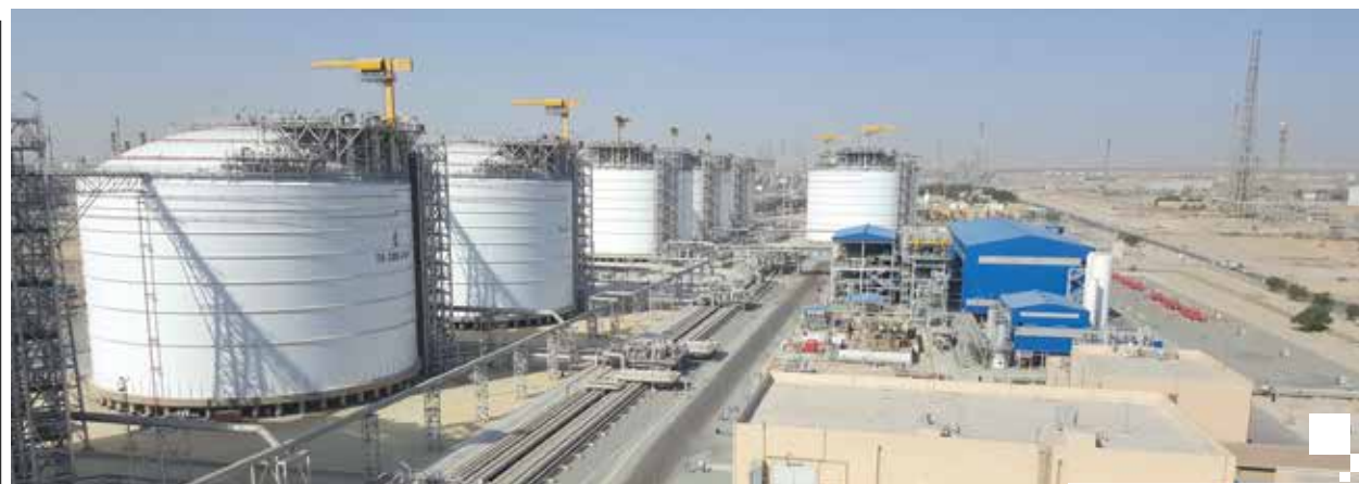
LPG North Tank Farm Project
