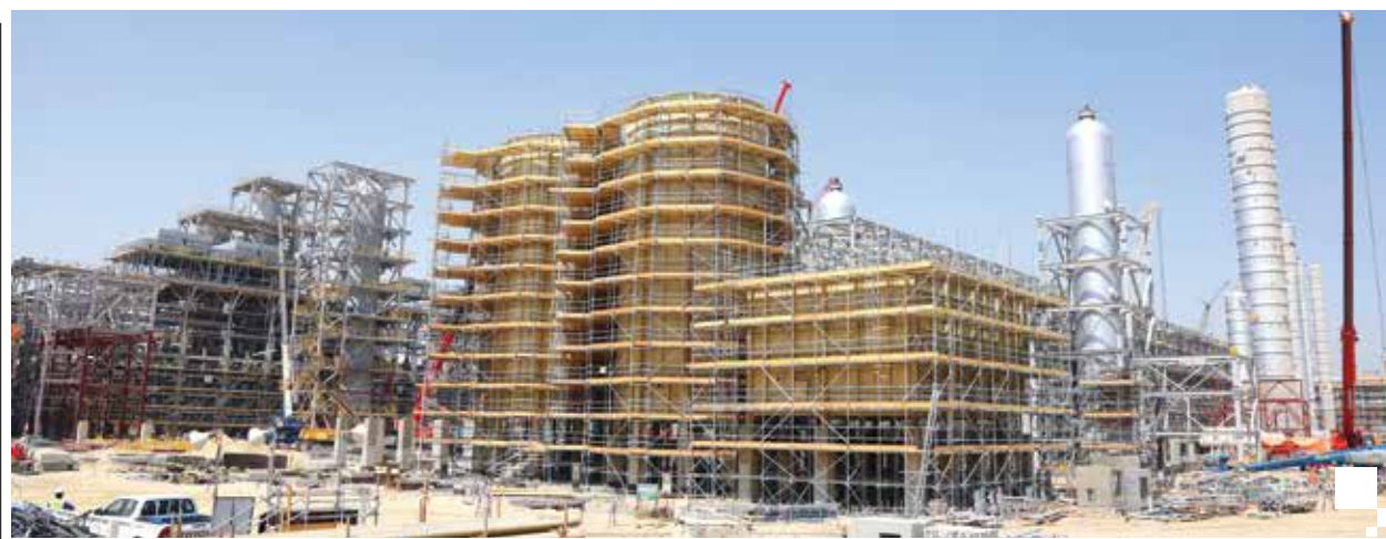
Construction works at CFP
