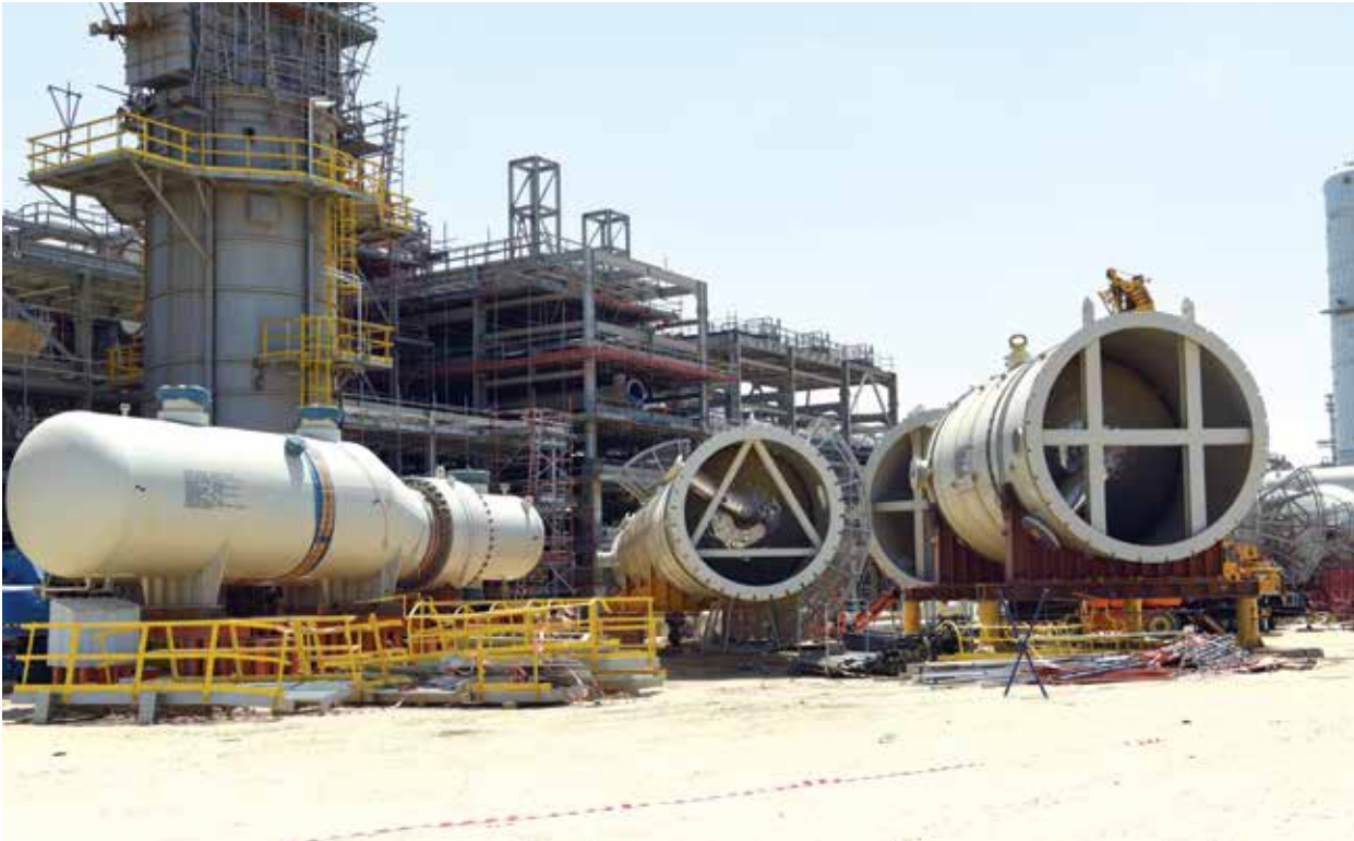
Gas Train Project - 5
