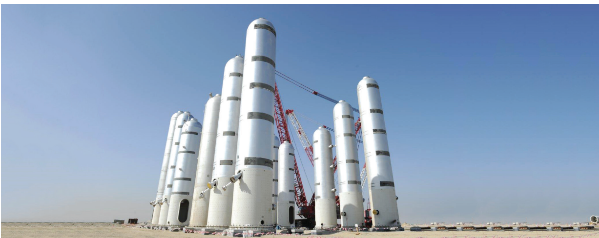
Installation of Reactors at ZOR Project
