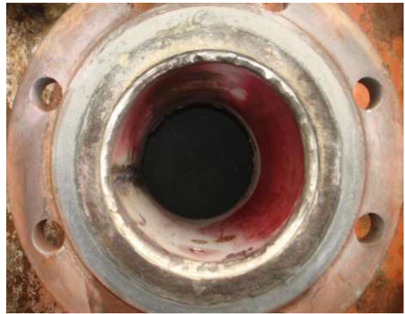
Sleeve installed on the nozzle ID
