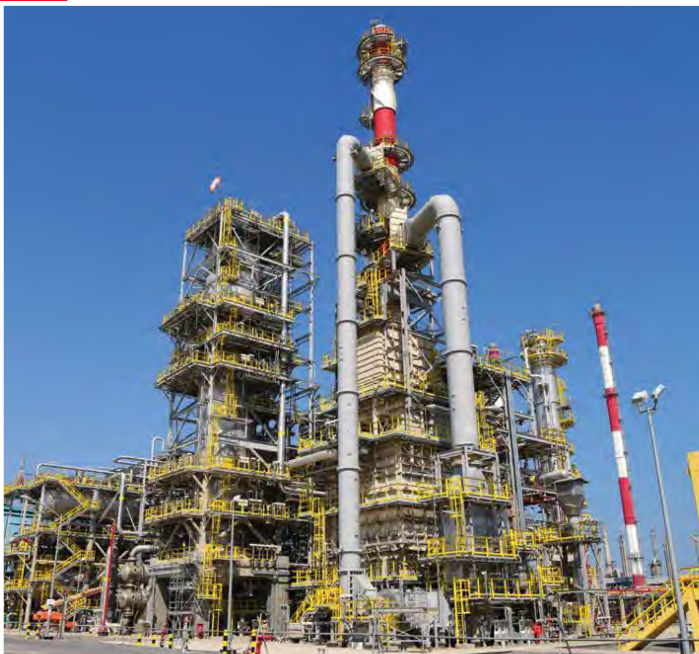
Diesel Unit 216 produces ULSD
